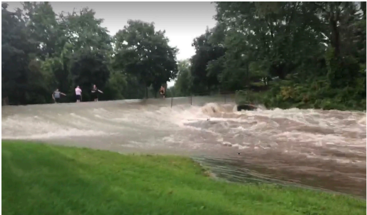
Looking NE at Lancaster Lane and culvert outlet ends – August 20, 2018
