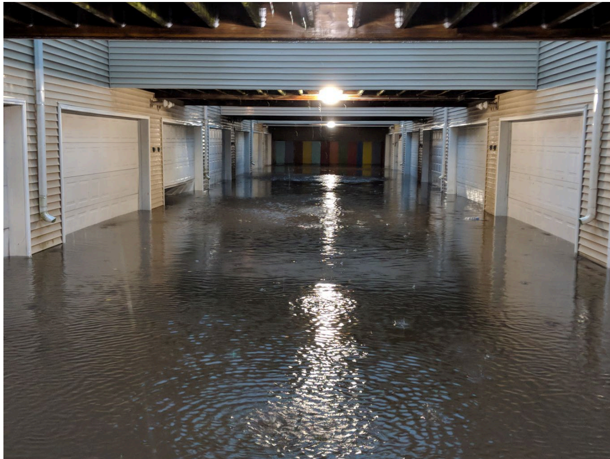
Looking west into underground parking at McKenna Rowhouses – August 20, 2018
